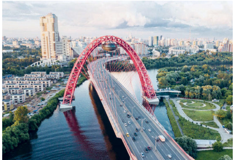
The Zhivopisny Bridge is the first cable-stayed bridge over the Moskva River
